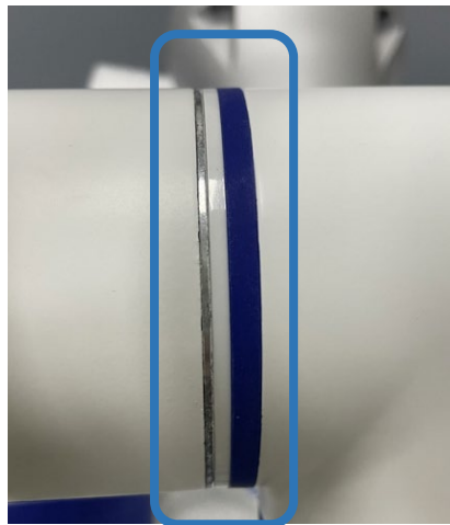
Figure 3-5 Install supporting rings and rubber rings
