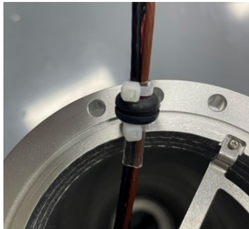
Figure 3-21 Tie the wire
